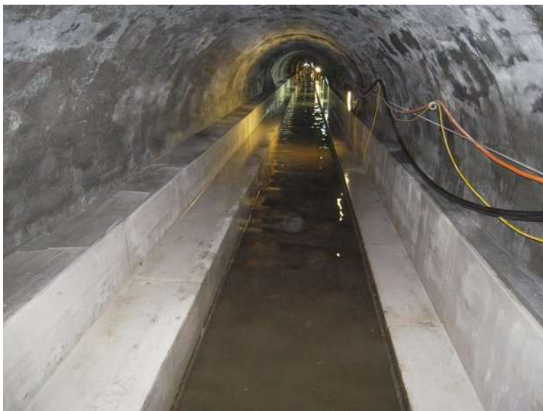
Figure 3 Heat exchangers in a sewage line by Kasag Swiss AB [24]
